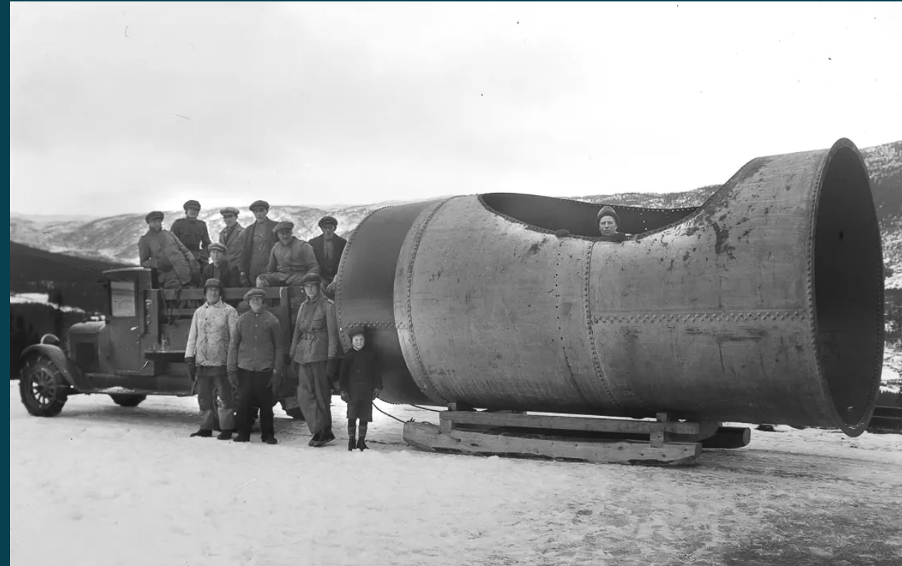
Truck and penstock – Hol development, Hallingdal 1952
