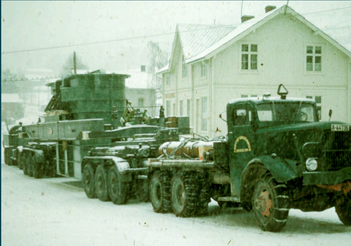
Tractor and transformer – Hemsil development, Hallingdal 1959
